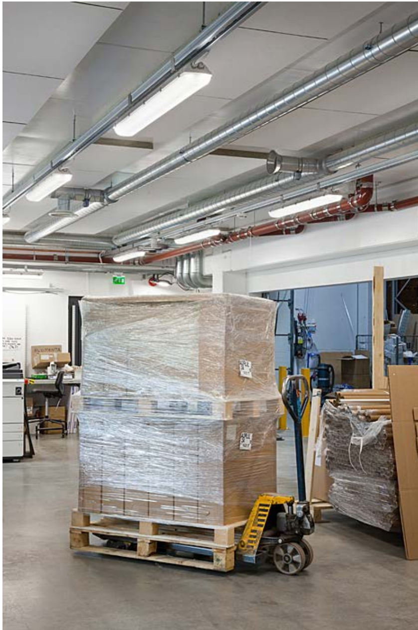
Airam warehouse and logistics.
